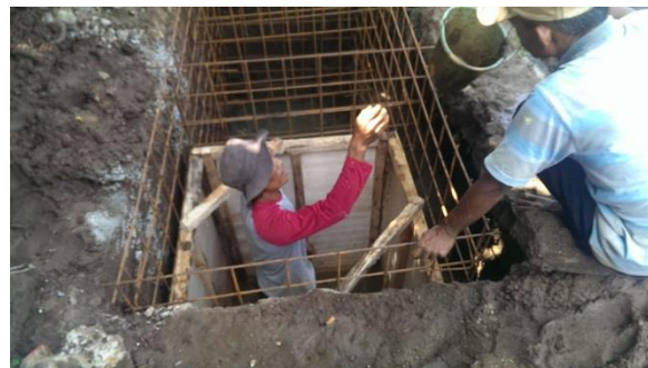
Gambar 6 Pengecoran dinding septic tank
