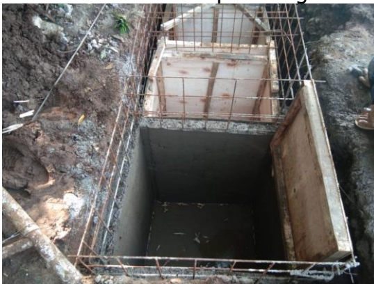
Gambar 6 Pengecoran dinding septic tank
