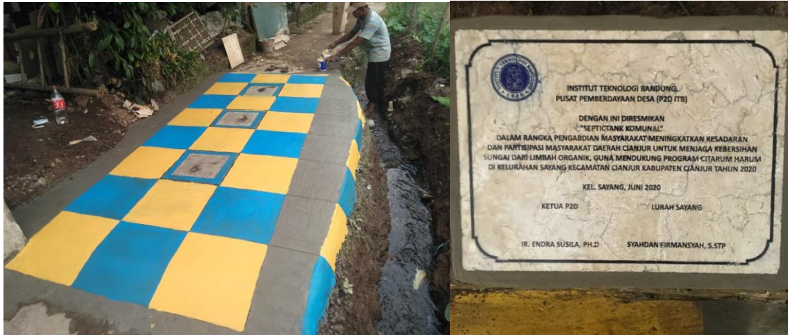
Gambar 10 Septic tank umum
